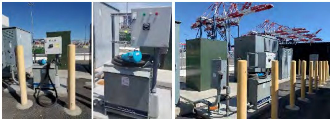
Figure 16: TransPower EV charging station at LBCT to support the battery-electric Kalmar yard tractor
