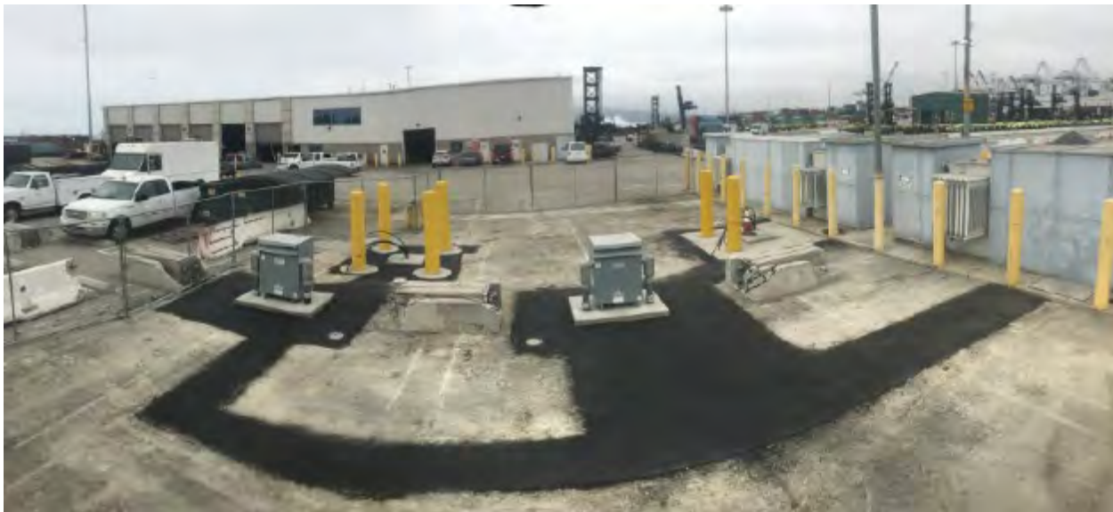
Figure 17: Stub-out completion at SSA Marine for the two BYD chargers to support the top handlers
