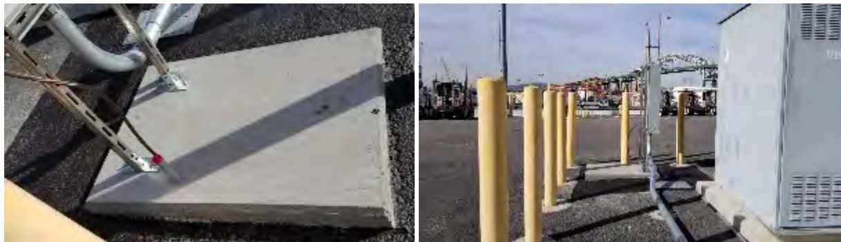
Figure 14: Infrastructure completion, ahead of delivery, at LBCT to prepare for the installation of the TransPower unit, including a closeup of the concrete pad and stub-out (left) and the same pad showing the breaker and its proximity to the safety bollards and necessary transformer (right)
