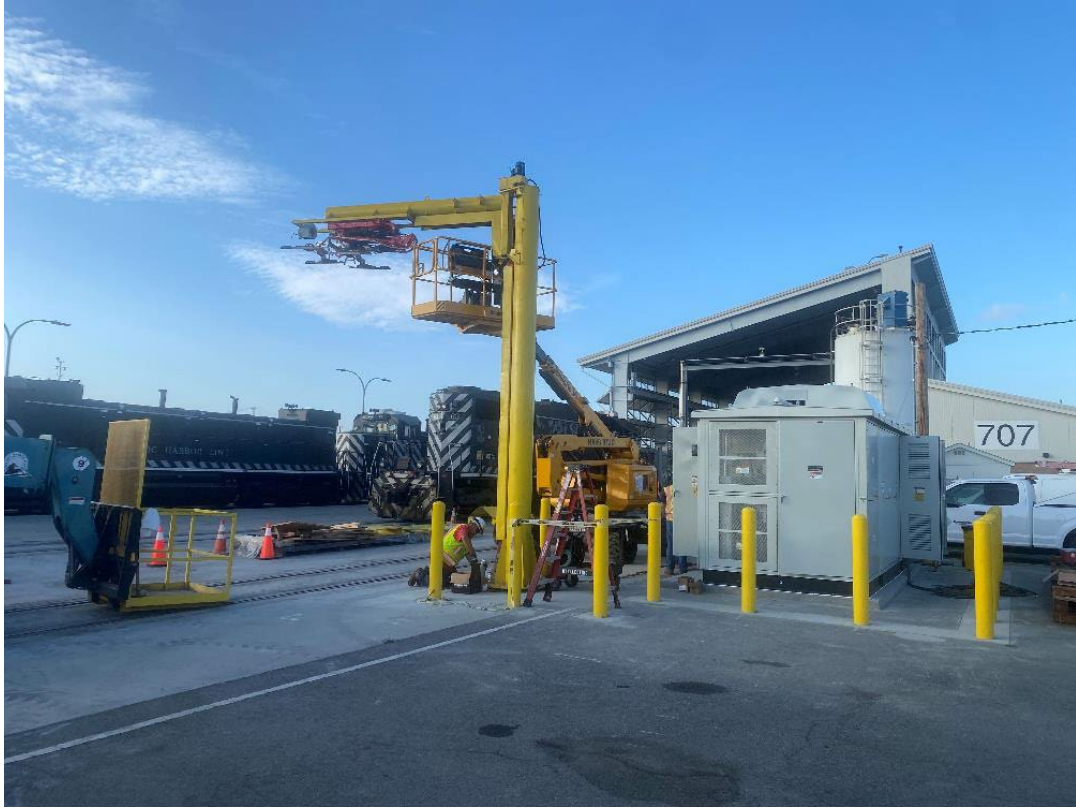
Figure 4: PHL Locomotive Charging System Under Construction
