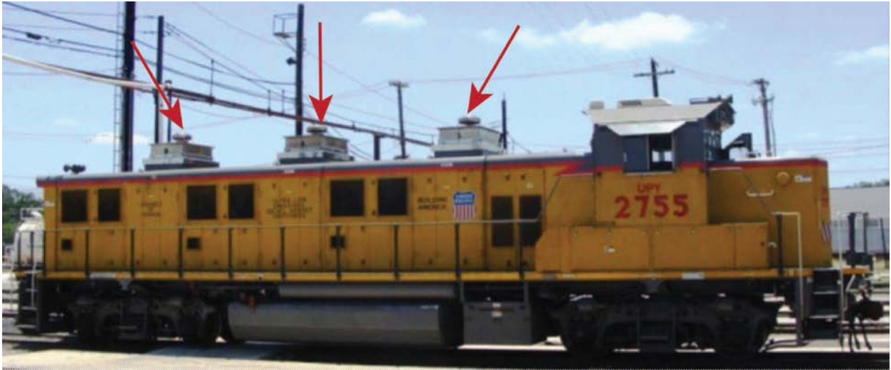
Figure 2.2: Johnson Matthey System Fully Installed on all three Gensets of UPY-2755
